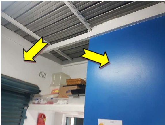
Photo 9. Interior, canteen, throughout, walls – suspected lead-containing white and dark blue upper coloured paint systems.
