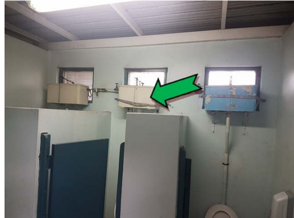
Photo 2. Interior, throughout, cisterns – non asbestos-containing moulded fibre cement.
